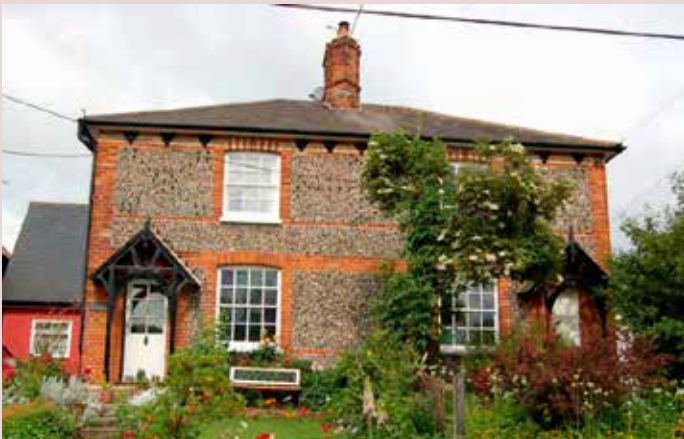
▲ Flint Cottages with red brick quoins on the High Street at Widdington.
