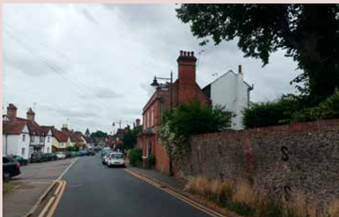
▲ Sense of arrival entering East on Lower Street through varied roofscapes and animated landscape features.
