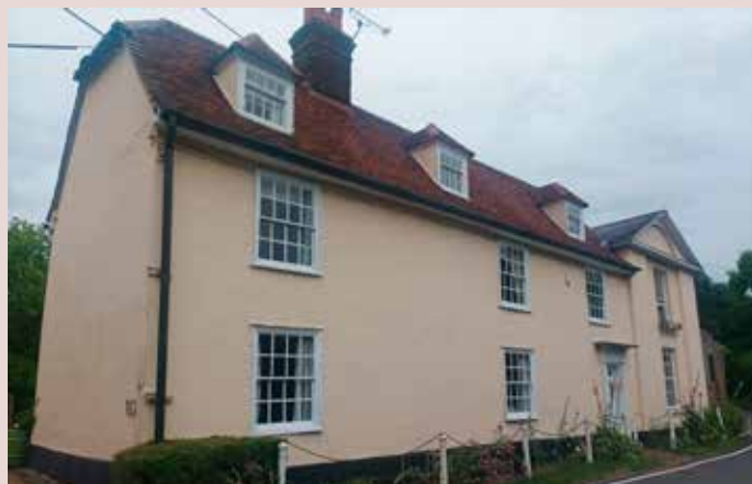
▲ Peg tiled roof, sash, pilasters and dormer windows with soft boundary treatment at B1039, Wendens Ambo.
