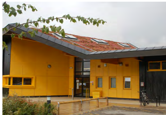
▲ Green roof in Broughton, Milton Keynes is an effective strategy to reduce surface runoff and recycle rainwater.
