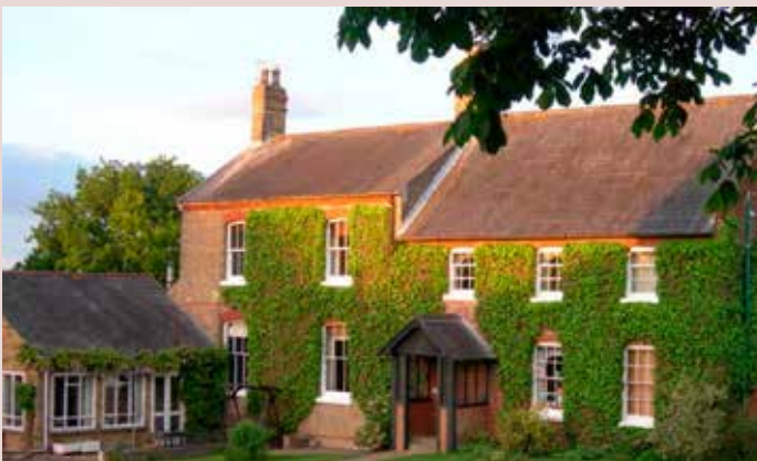
▲ Ivy clad 19th Century Farmhouse on Friars Lane contains strong farmland views in a natural rural setting.
