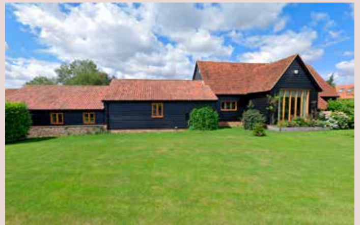
▲ Local farmstead vernacular (black weatherboarding, peg tiled roof and flint wall) in Baconend Green.
