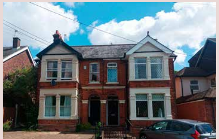
▲ Edwardian paired semi-detached houses with red brick and arched doorways on Station Road.
