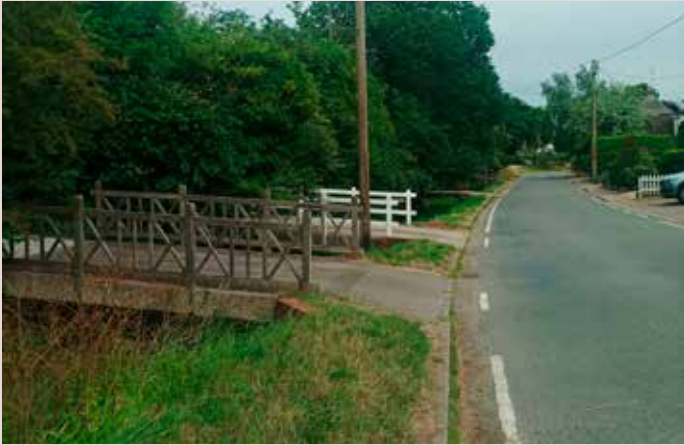
▲ Bridges to homes over swales and green verges on the Main Street, Arkesden.
