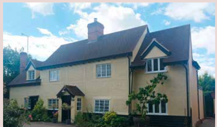
▲ Peg tiled roof, pargetting, dormer windows, central chimney and black weatherboarding Dunmow Road, Takeley.
