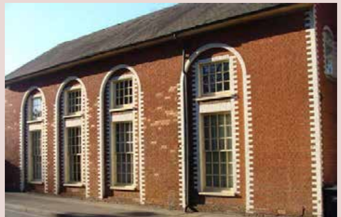
▲ Arched windows and flint wall positively addressing London Road.
