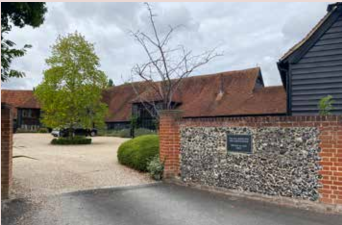
▲ Black weatherboarded barn conversion with dormers, shared courtyard and stone wall boundary at Hall Barn and Garden House.
