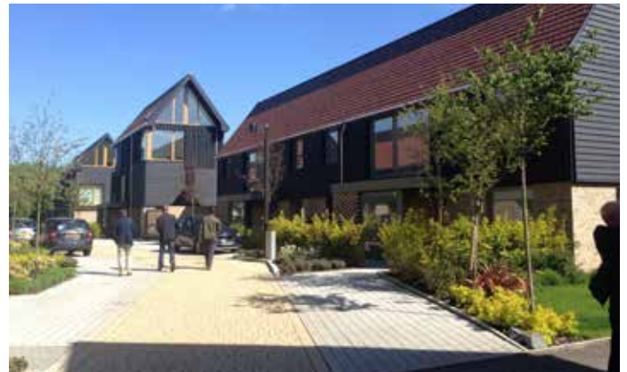
▲ Lanes within higher density development use informal landscaping and clearly define parking bays.
