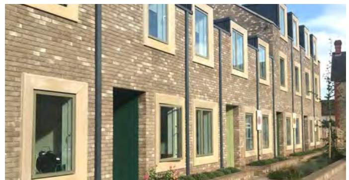
▲ Homes in Temple Gardens maximise thermal efficiency through glazing and southern orientation.
