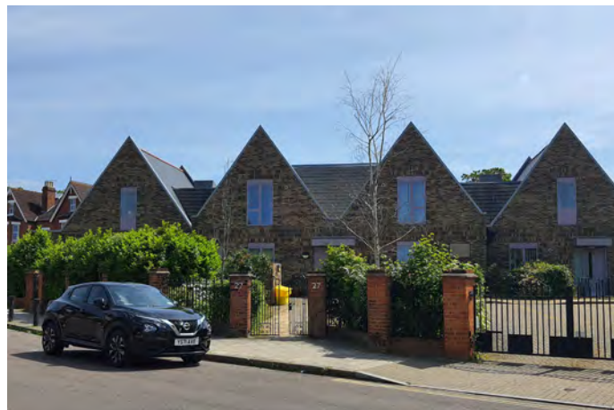
▲ Thrale Almshouses in Streatham - refurbishment and extension of existing almshouses set around a secure landscaped courtyard. Almshouse models work for young families, young people and older persons, providing community and safe and secure housing with a sense of purpose.
