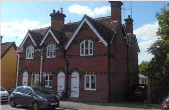
▲ Pleasing terrace of nineteenth century houses with prominent chimneys, elaborate decorative brickwork and patterned bargeboards.
