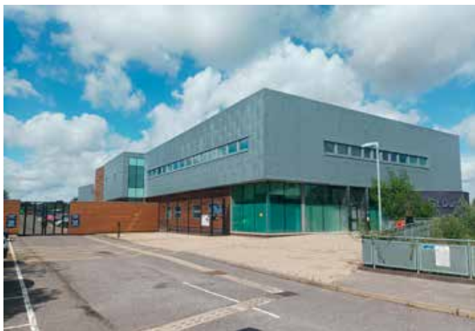
▲ Police station in Great Dunmow uses active frontage at the ground floor and has a clear, well-lit and welcoming entrance.
