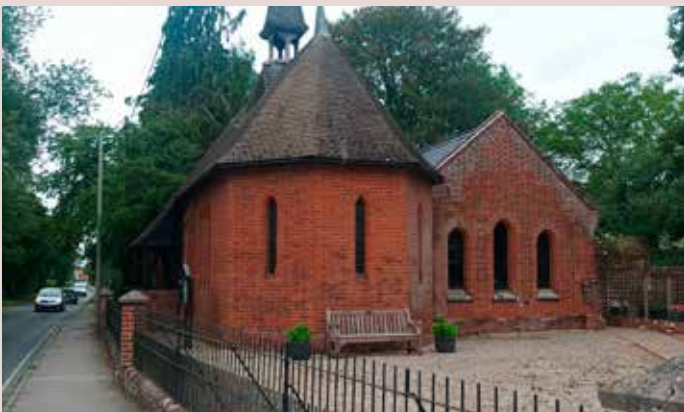
▲ St. James chapel in Swards End comprises of a semi-hexagonal apse and fourlegged belfry with fleche.
