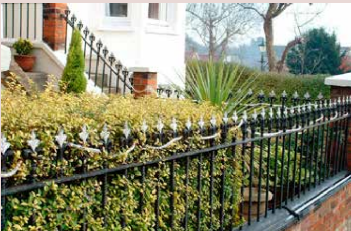
▲ 19th Century railings form an important feature in the defensible space of homes in Stansted Mountfitchet.
