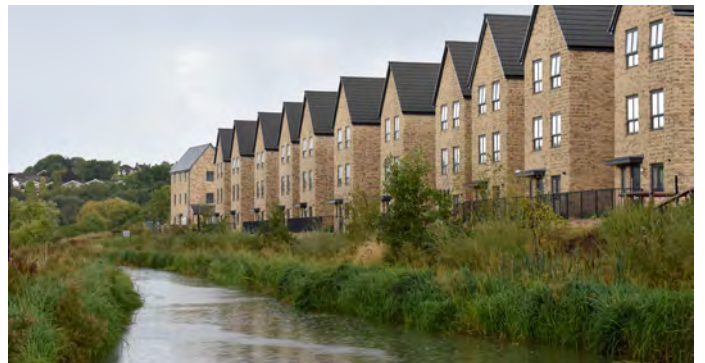
▲ In Wichelstow the natural character of the river has been integrated into the development. Green banks provide space for habitats to thrive.
