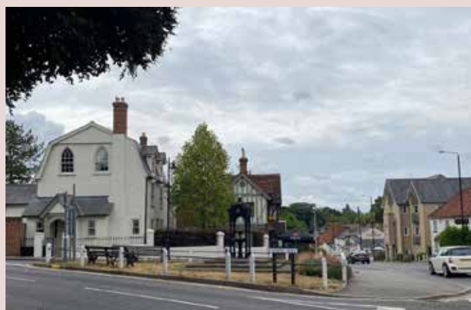
▲ Central green space with landmark on Chapel Hill creates a gateway into the town centre.
