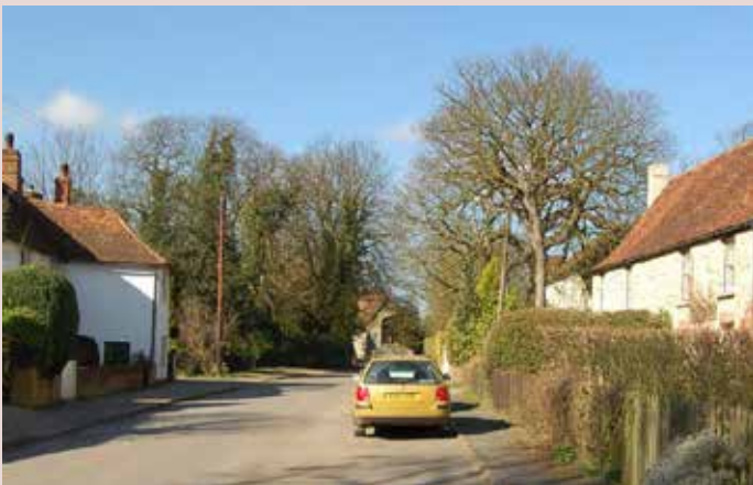
▲ Historic buildings frame a view to the west on Church Street in Henham.
