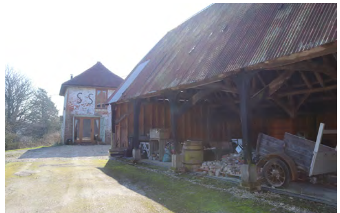
▲ Retrofitted heritage assets enhance the farmstead narrative.
