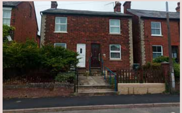
▲ Red brick Victorian terraces with exterior chimneys, Ashdon Road.
