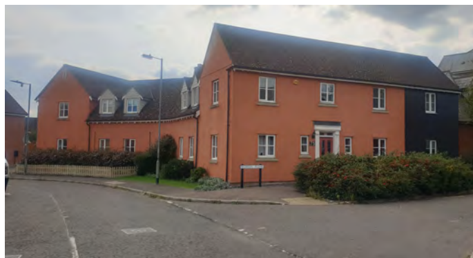
▲ Joined buildings at Flich Green create a compact development and make reference to local vernacular.
