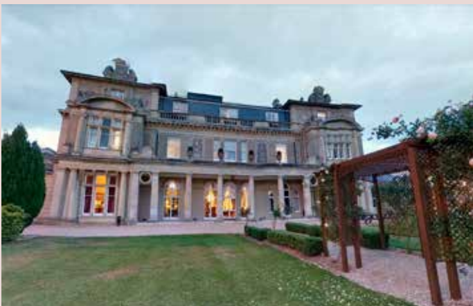
▲ Three storeyed manor house at Down Hall Hatfield Heath. Pillars and statues.
