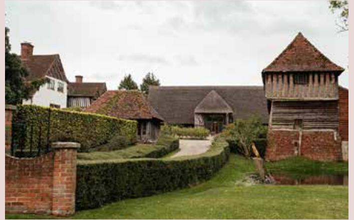
▲ Colville Hall in Uttlesford with Thatched roofs, timber frames, and jettying.
