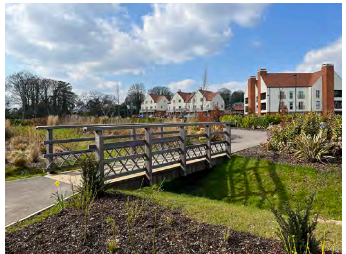
▲ A bridge facilitating access over a planted swale that has been successfully integrated into a local open space.
