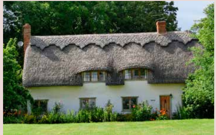
▲ Dormer windows on the 17th Century thatched cottage in Takeley.
