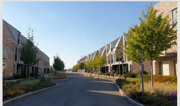
▲ Rich landscapes are integrated within the streets and limit driveways to maximise connectivity
