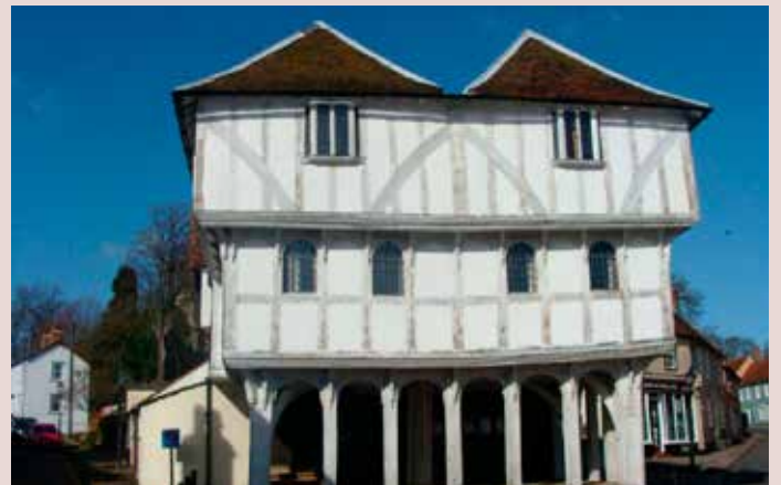
▲ Grade I listed Guildhall in Thaxted, ground floor forms open flagged market house with open timber ceiling, and heavy cross beams.
