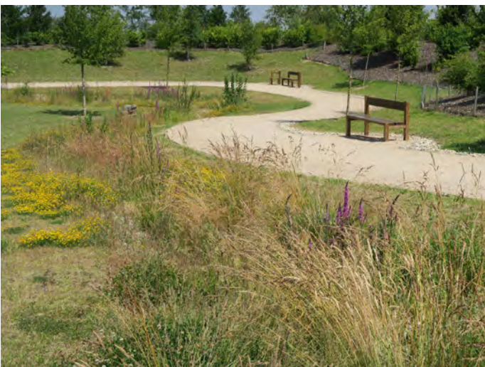
▲ A linear swale with biodiverse planting integrated into a local park space.
