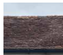
Peg tiled roof
