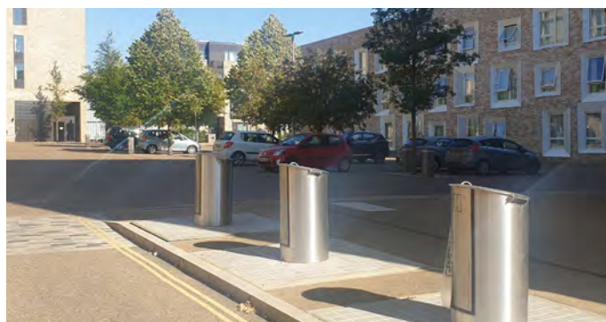
▲ Communal waste points in Eddington, Cambridge, are effectively integrated into the street scene. Communal waste points allow for a designated service route in the development.
