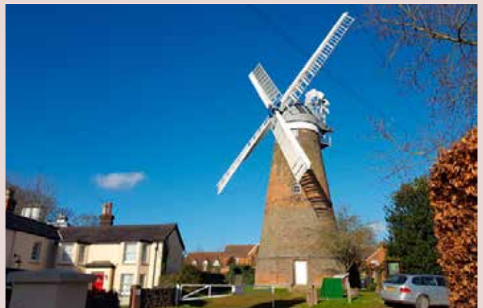
▲ Windmill typologies and materials influence the built form Stansted Mountfitchet and elsewhere in Uttlesford.
