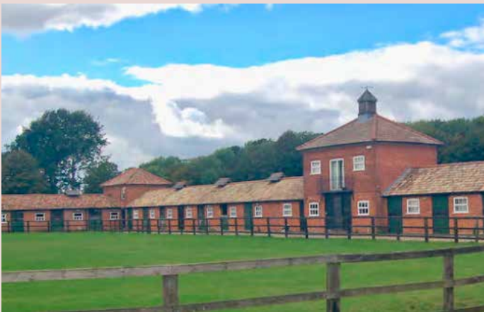
▲ Individual single-storey stables at Brookend Farm Stables. Central two-storey block - built with red brick, projecting wings and gabled tile roof.
