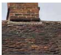
Peg tiled roof
