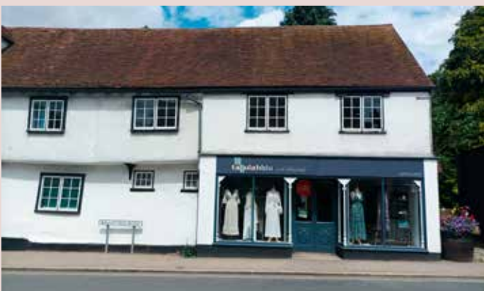
▲ Modern shopfront design integrated into historic built form - Braintree Road, Felsted.
