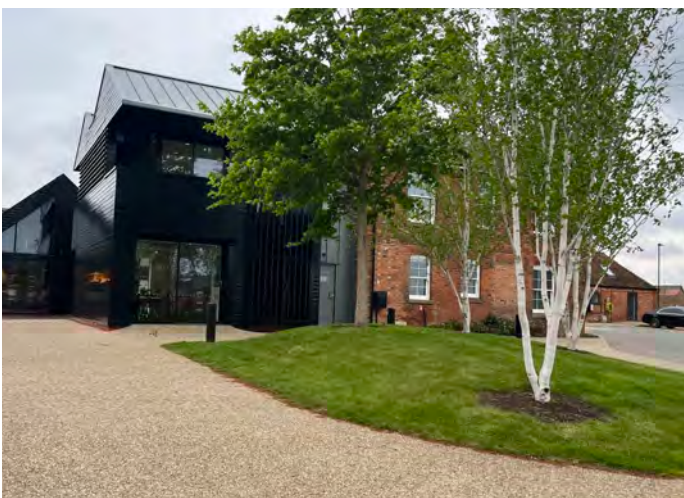
▲ Existing barn converted and extended to provide a visitor centre at Houlton, Rugby alongside community uses and a cafe.
