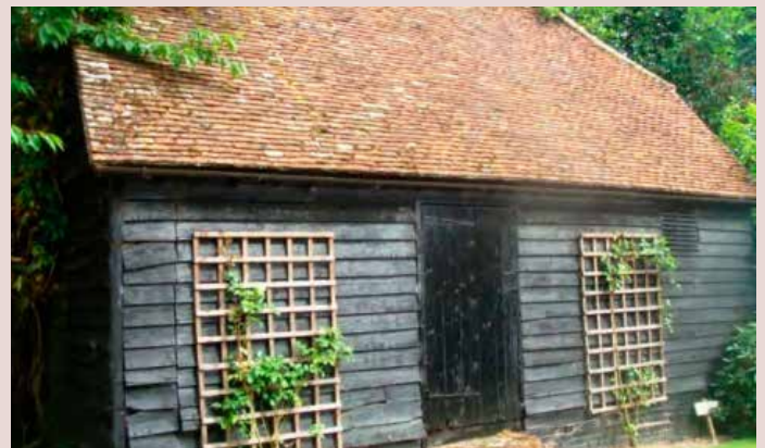
▲ Black weatherboarded barn with peg tiled roof demonstrates character at the smallest scale in Elmdon.
