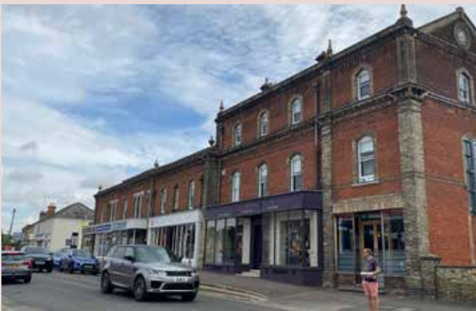
▲ Historic red brick with eave detailing integrating Cambridge Road shops.
