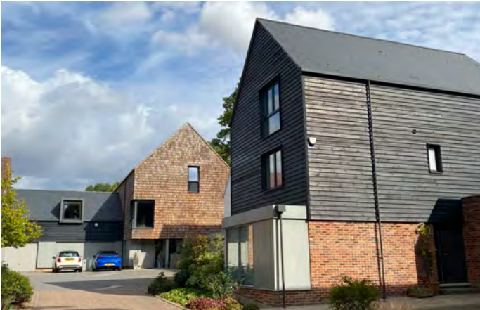
▲ The Avenue, Saffron Walden provides residents with comfortable living conditions and generous private/shared external amenity space.
