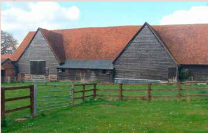
▲ Grade II listed Bury Farm Barn, Felsted, with a restored weatherboarded timber framed and Queen post roof structure.
