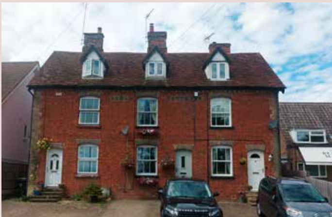
▲ Dormer windows and central stack chimneys create strong character for red brick terraces.
