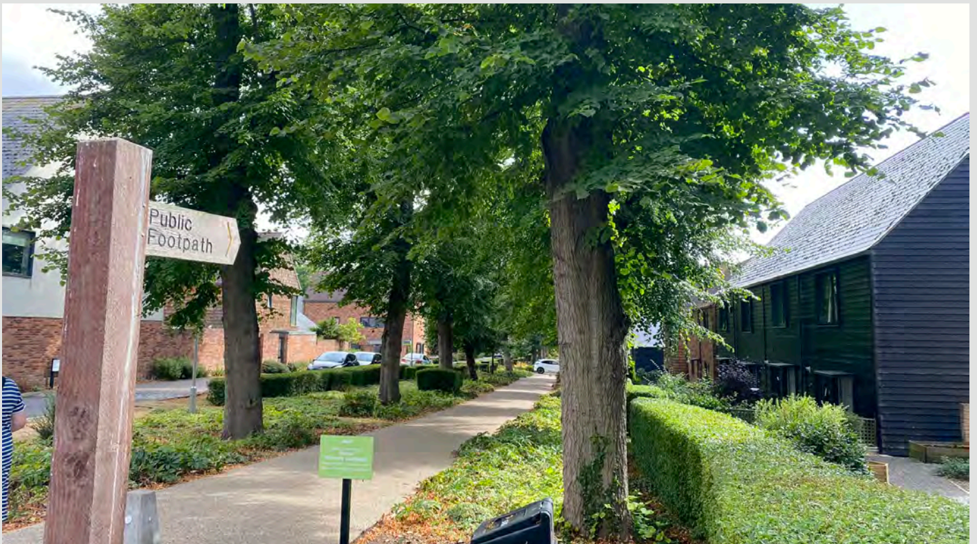
▲ Segregated pedestrian and cycle route created within the place-defining lime-tree avenue. The path is well-overlooked and integrated with homes on both sides bringing residents closer to nature.
