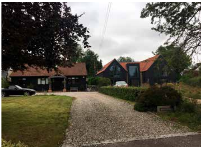
▲ Use of black timber referencing surrounding farm buildings in Duddenhoe End.
