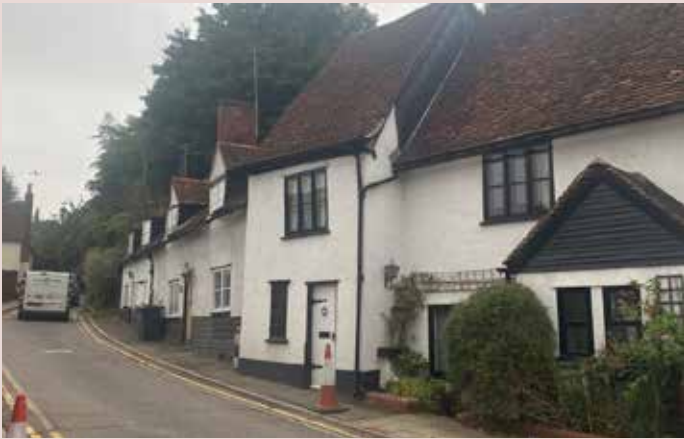
▲ Consistent Timber framed terraces on Grove Hill with minor differences creating a coherent sense of character without repetition.
