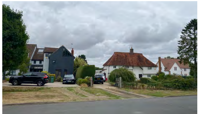
▲ Broken building line with gaps between buildings and greater setback in Stansted Mountfitchet.
