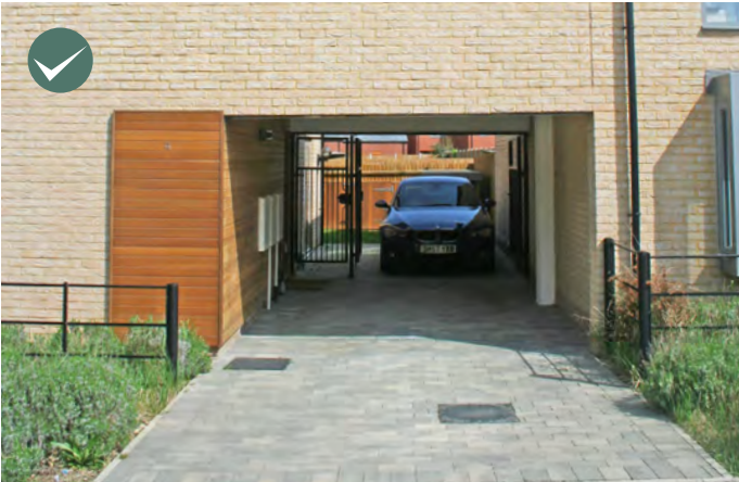
▲ Car parking concealed on plot through the integration of a car port.
