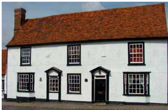
▲ The Bell in Great Easton, a former public house dating back to the 15th century, comprises of a timber framed building with plastered and pargetting facades.
