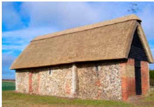
▲ Brick-and-flint building with weatherboarding and thatched roof in Wicken Bonhunt.
