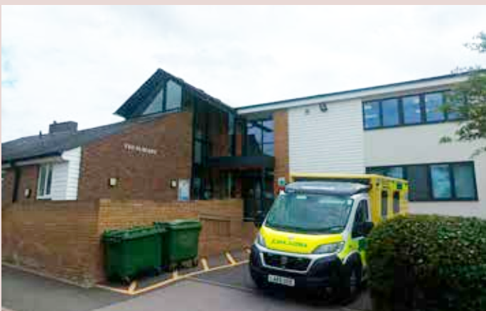
▲ Thaxted Surgery uses varied roof forms and pitches to compliment the character of the town.
