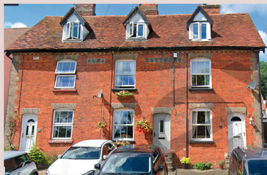
▲ Dormer windows and central stack chimneys create strong character for red brick terraces
