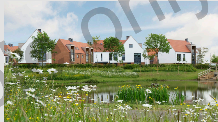
▲ Central pond provides a safe environment for breeding birds and wildlife whilst forming a key part of the sustainable drainage system and an attractive landscape feature, designed without a need for fenced edges
