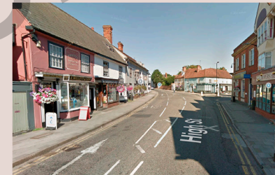
▲ Strong continuous built form frontage reinforces hierarchy of character and use along High Street, Great Dunmow
